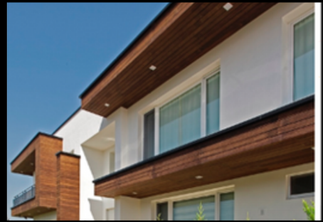
MOSO® Tongue & Groove boards create a dense, continuous installed surface.
